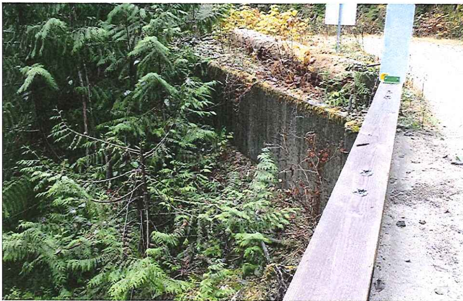
CK2112 Right Wingwall Downstream
