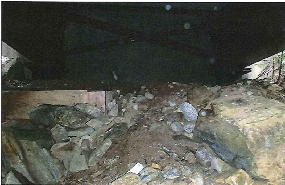
CK2112 Left Abutment
