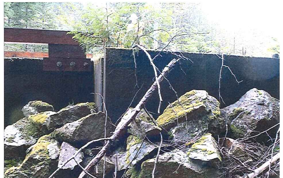
CK2112 Right Wingwall Upstream
