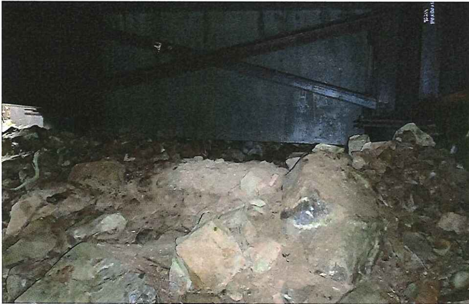
CK2112 Right Abutment
